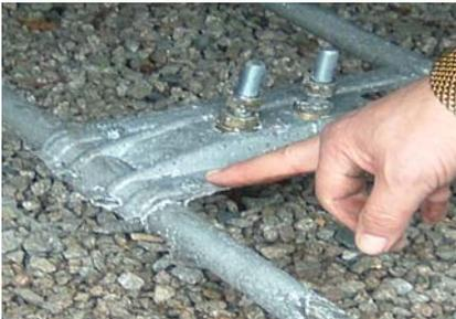
Undo the small nuts and slide the side bracket along.
